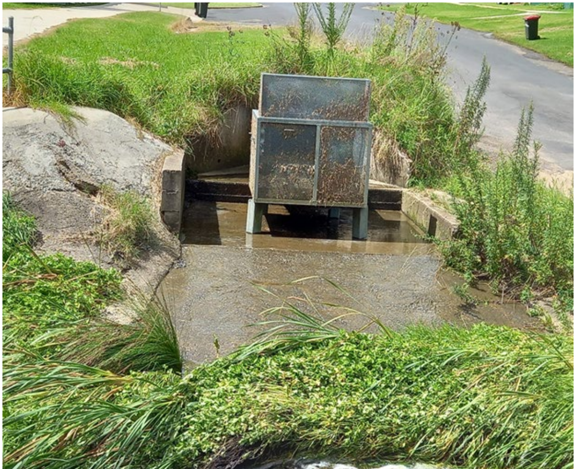
Figure 3.12.2: Gross Pollutant trap in “Excellent” condition
